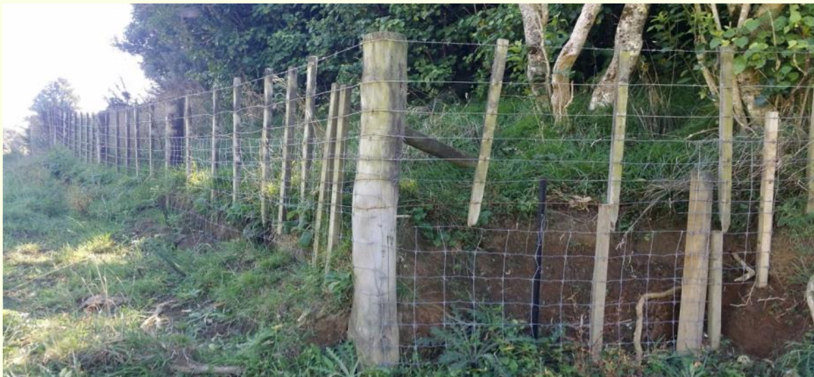
Fence repairs were carried out in 2015
